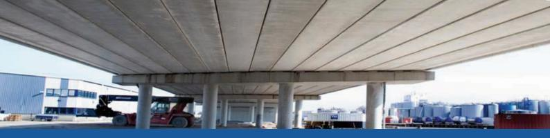
Haitsma Beton's long beams, whose enormous span (our tensioning device is 90 m long!) renders intermediate pillars obsolete, offer new perspectives for the construction of roads and waterways. These beams will enable you to reduce construction time for bridges and viaducts, as well as to guarantee improved access to both road and water transport.
